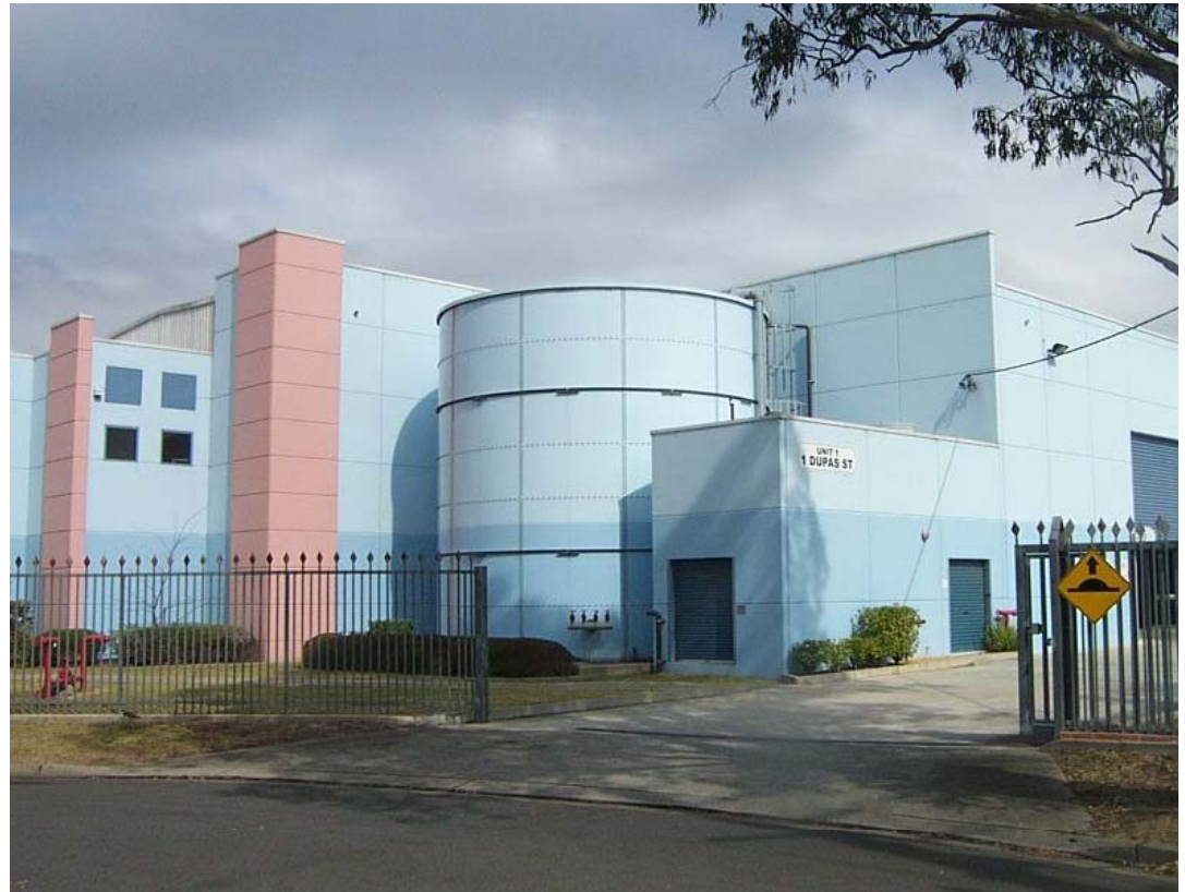
Photo Above: Completed tank constructed to fit into building's pre-existing structure.
