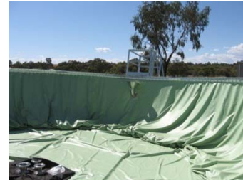
Photo Far Left: Tank Liner Application
