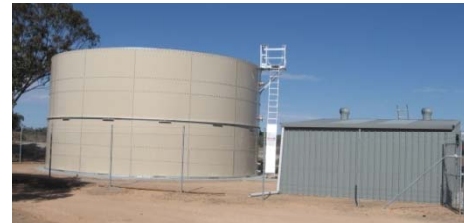
Photo Right: Completed TS600 Open Top Tank with Pump Shed visible
