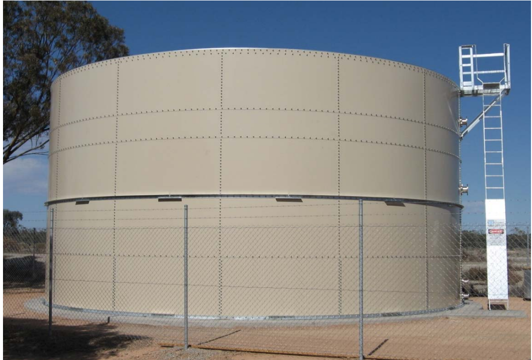
Photo Far Right: Ladder & Ladder Platform
